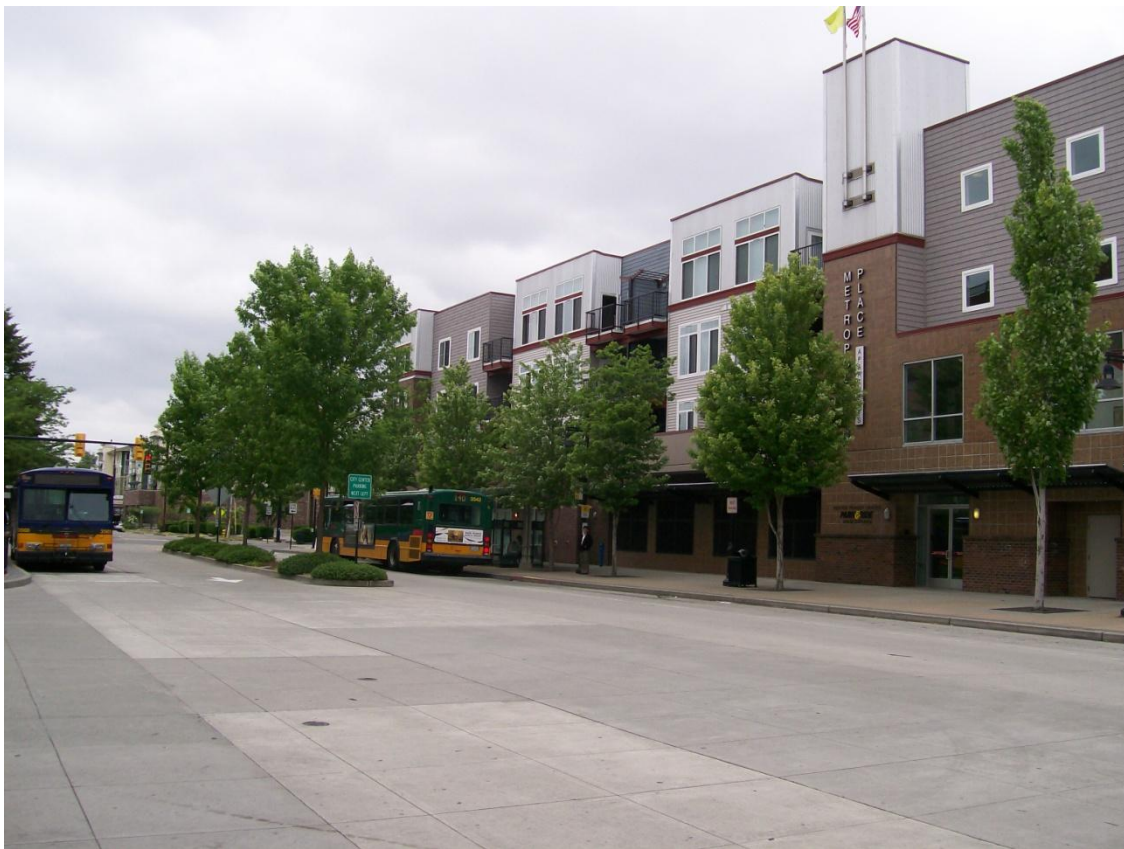
Figure 8. Metropolitan Place, Renton, April 2009.
